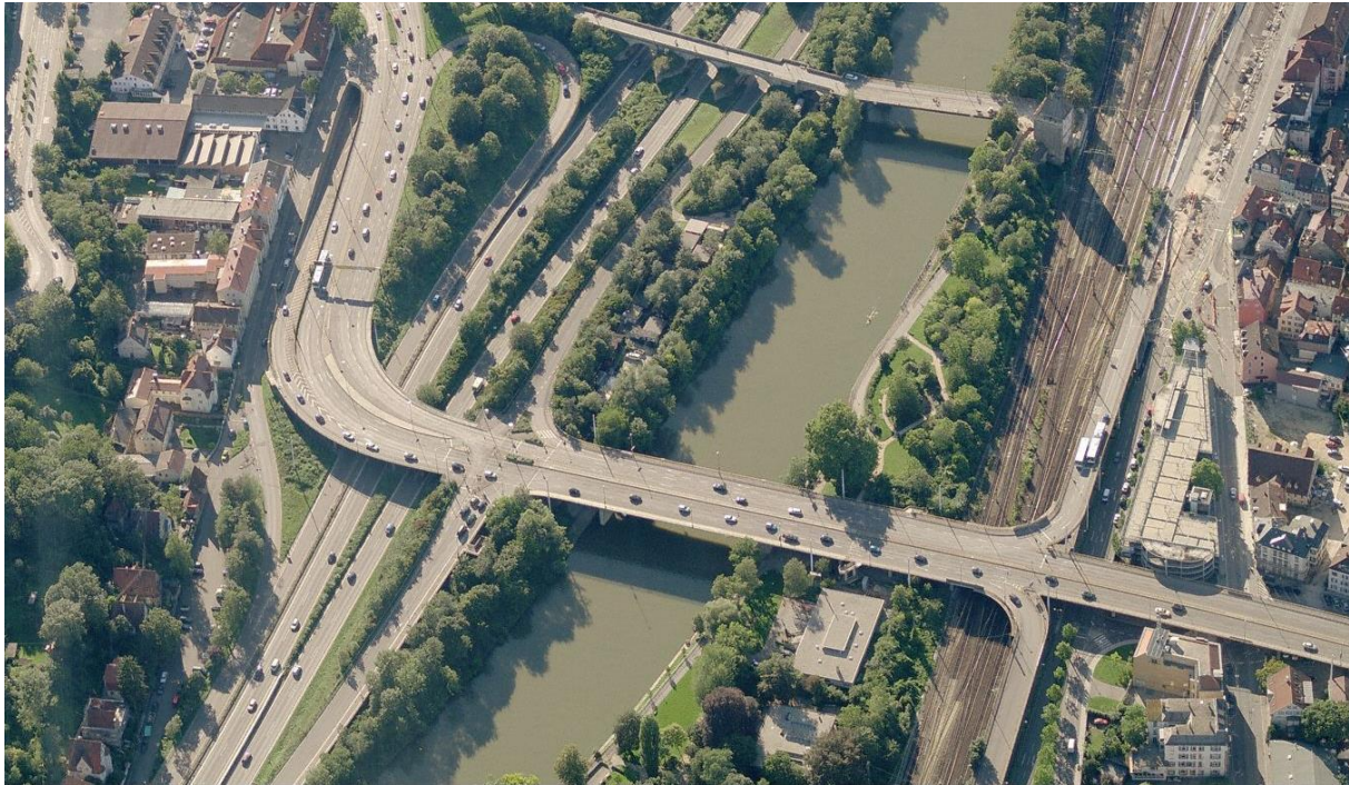
Fig. 3-6: Aerial image of Vogelsangbrücke Esslingen, Germany [source: maps.google.com]
