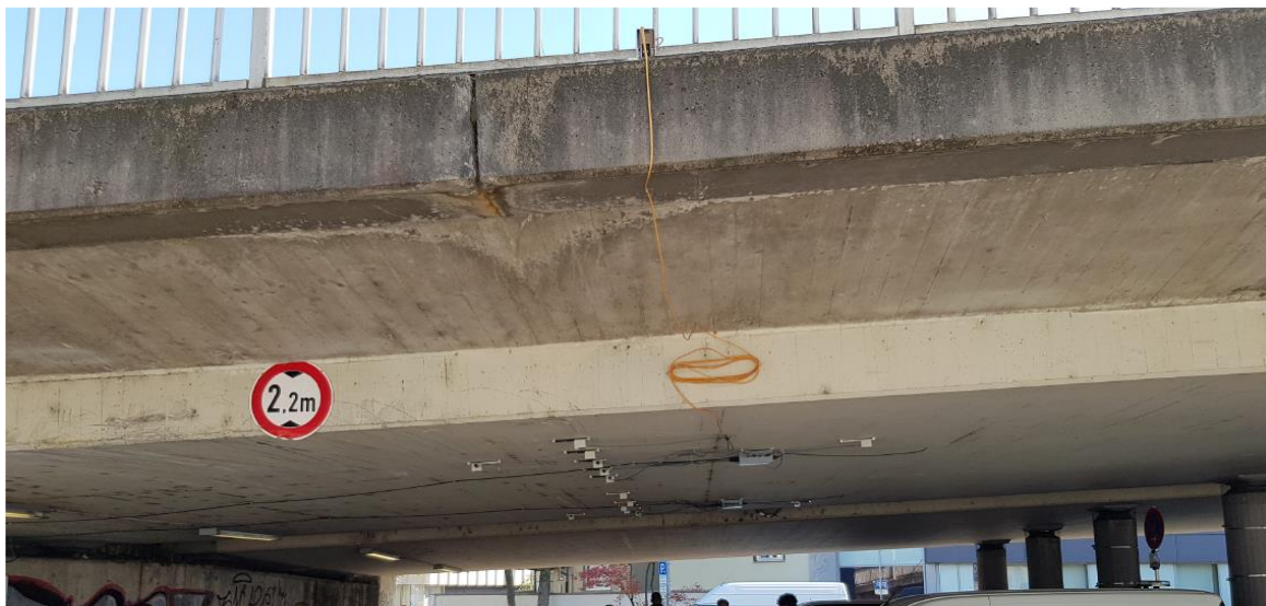
Fig. 3-9: View of the installed sensors
