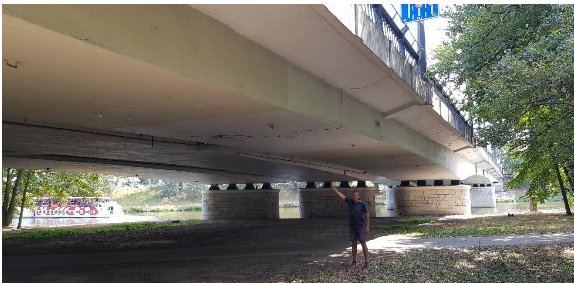
Fig. 3-1: Wonka bridge in Pardubice, Czech republic
